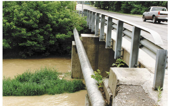
#2A Wax-Tape applied to bridge span, providing corrosion protection from road salt, physical damage and atmospheric corrosion.
