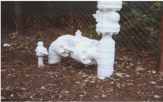
#2W Wax-Tape (white pigmented) easily applied to a difficult-to-protect wellhead. Note the complete conformity to the irregular surfaces.
