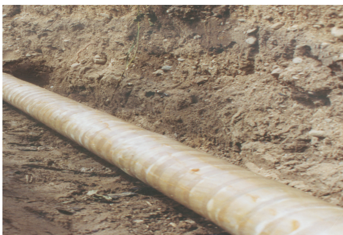
Section of 16" pipe reconditioned using #1 Wax-Tape.
