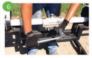
Torque nuts 50 to 70 ft/lbs to form a gasket seal. Do not over torque as it will not increase sealing ability and may cause plastic pipe failure.
