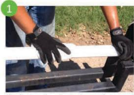
Check pipe diameter to insure that correct saddle is being installed and Thoroughly clean the pipe so surface is smooth and free of dirt and other debris.
