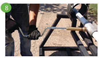
Tap through Corporation Stop using a VegaDrill for best results on plastic pipe.
