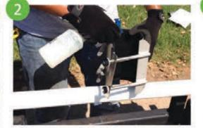
Lubricate of the gasket with a soap solution. For cold weather lubrication, ethylene glycol can be added to the soap solution to prevent freezing.
