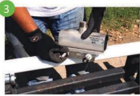
Loosen nuts until flush with top of studs, and place saddle around pipe.
